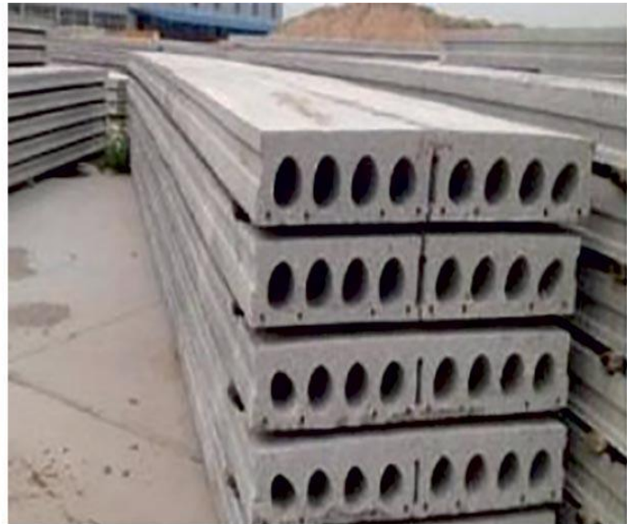
Figure 14: Pre-stressed precast system using hollow core slab
