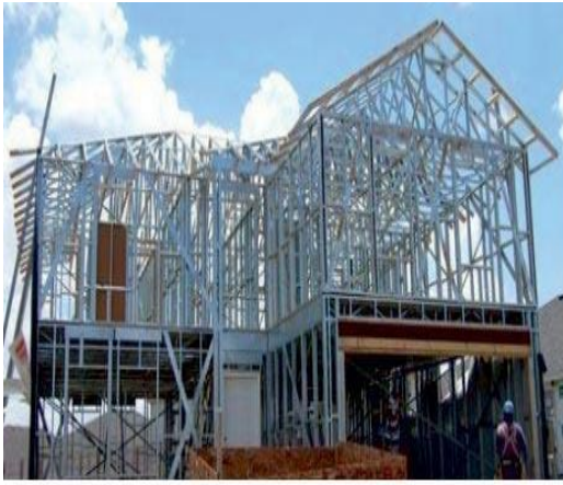
Figure 11: Light Gauge Steel Structural Systems Pod
