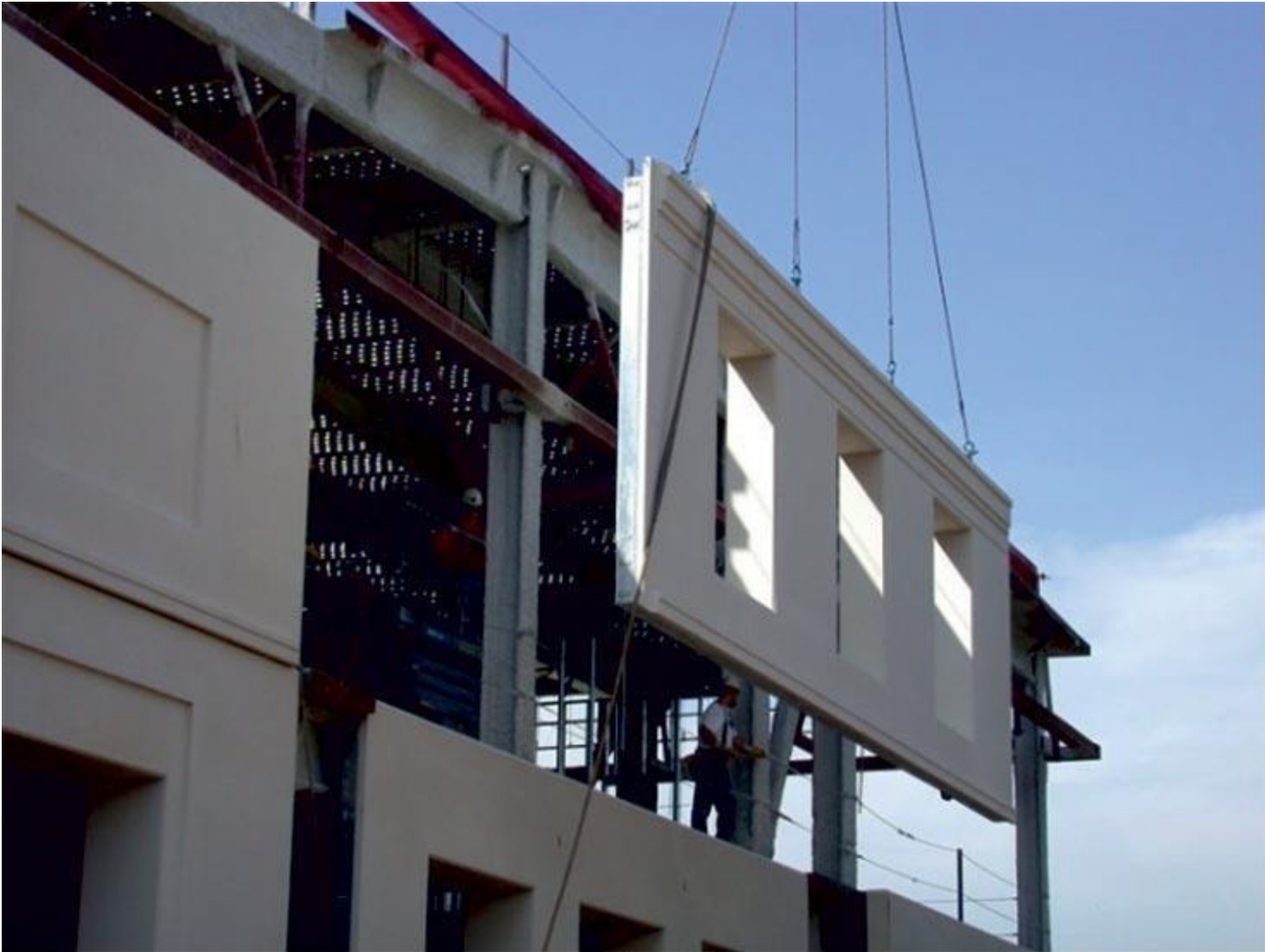
Figure 7: Panel prefab system
