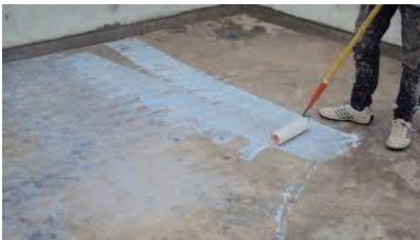
Fig.1. Application of Latex Bonding Agent
