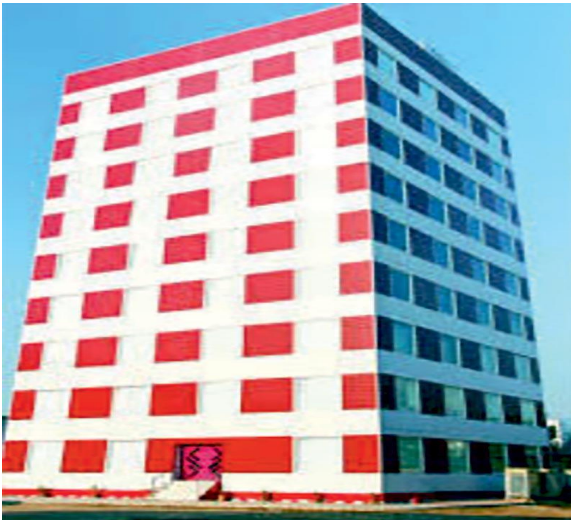
Figure 16: Factory made fast track modular building system
