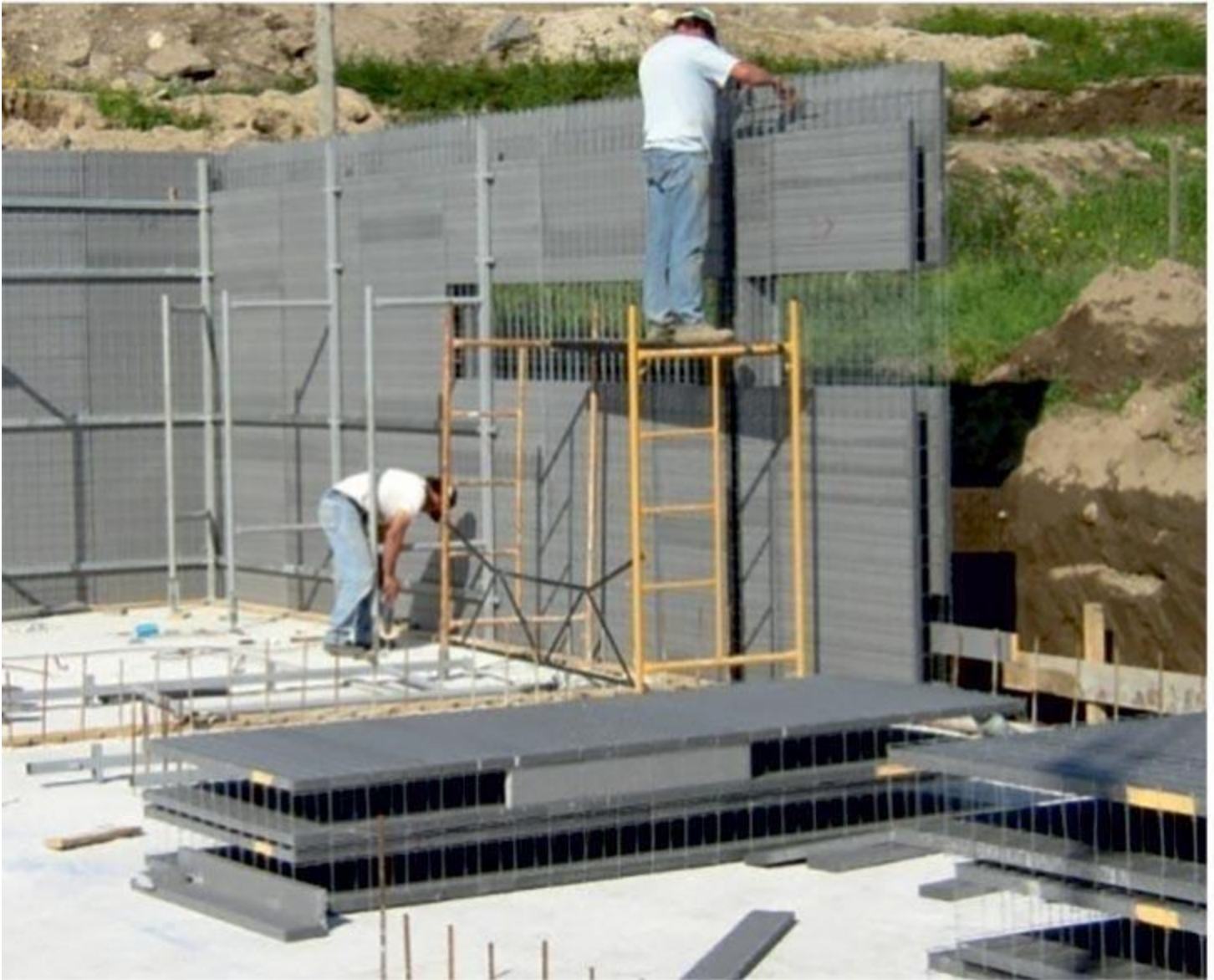
Figure 5: Construction of a wall with Sismo Technology
