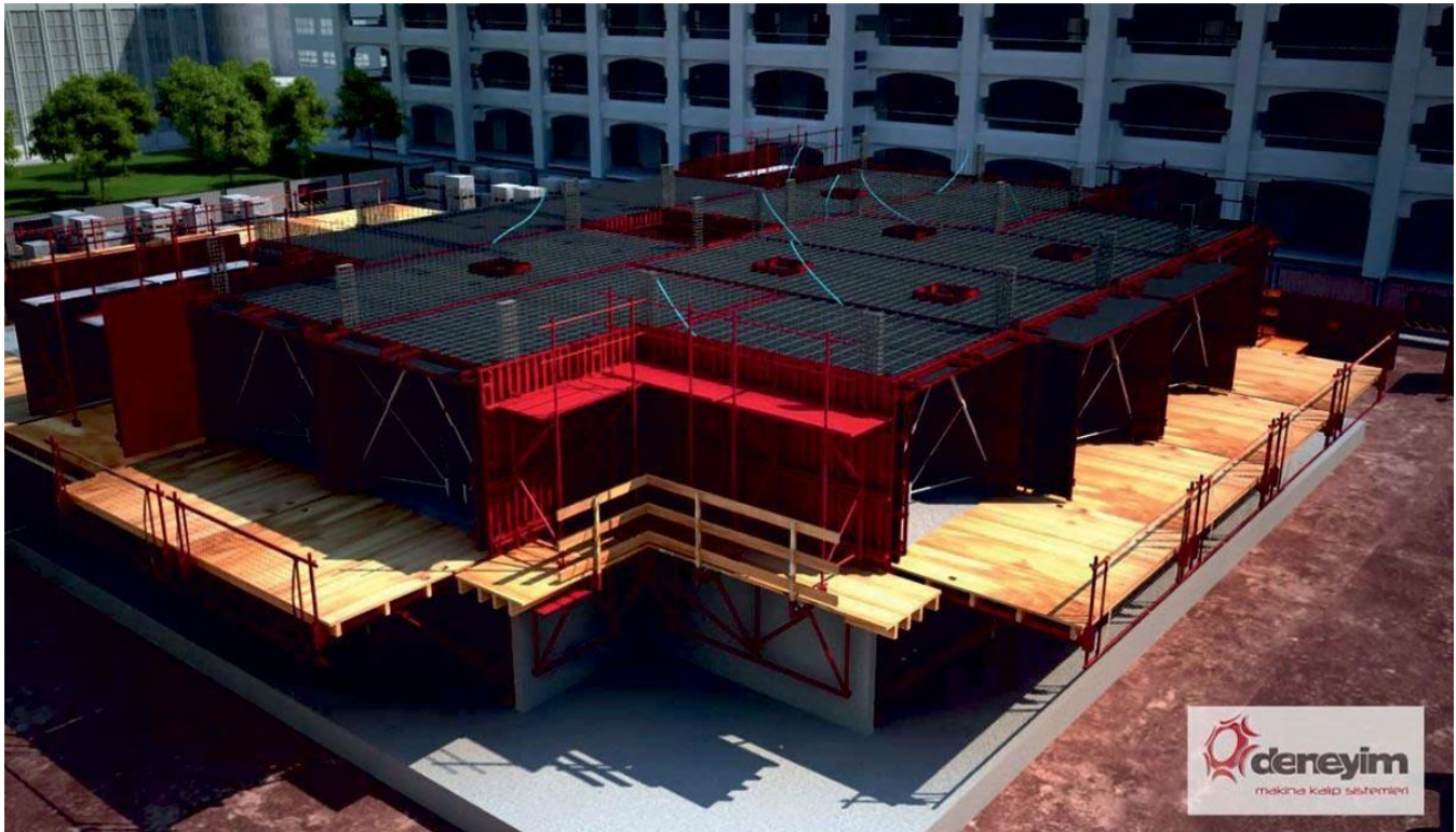
Figure 3: Cellular construction using modular tunnel
