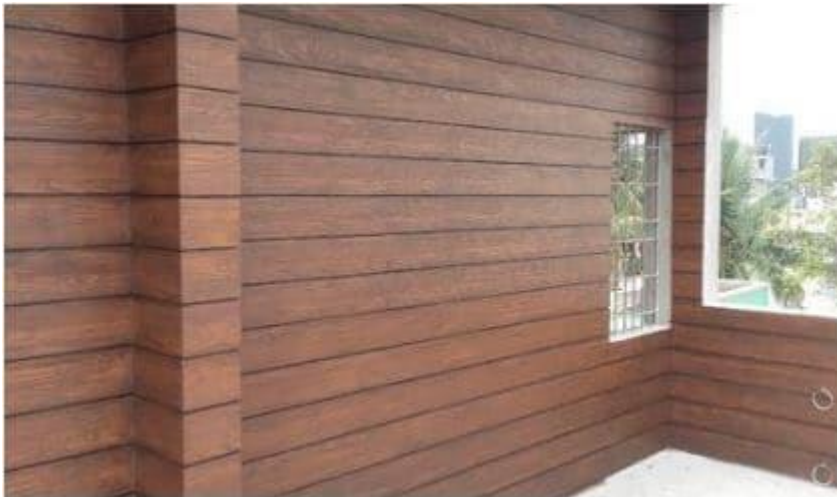
Fig.6. Fibre Cement Cladding
