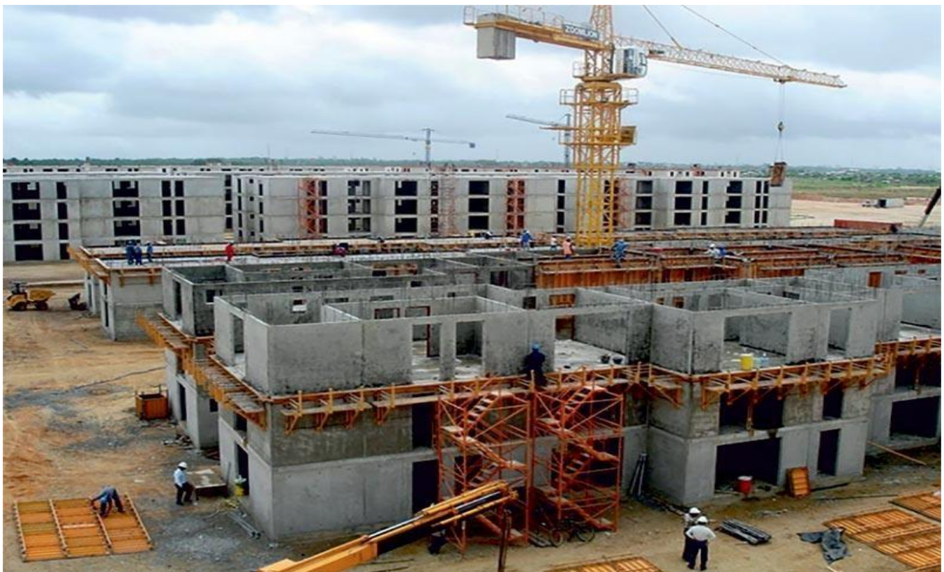
Figure 4: Kayson's formwork system construction
