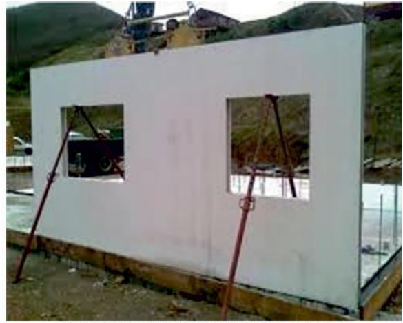
Figure 10: Glass fibre reinforced gypsum panel system
