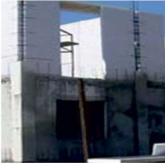
Figure 6: Expanded Polystyrene (EPS) core panel system
