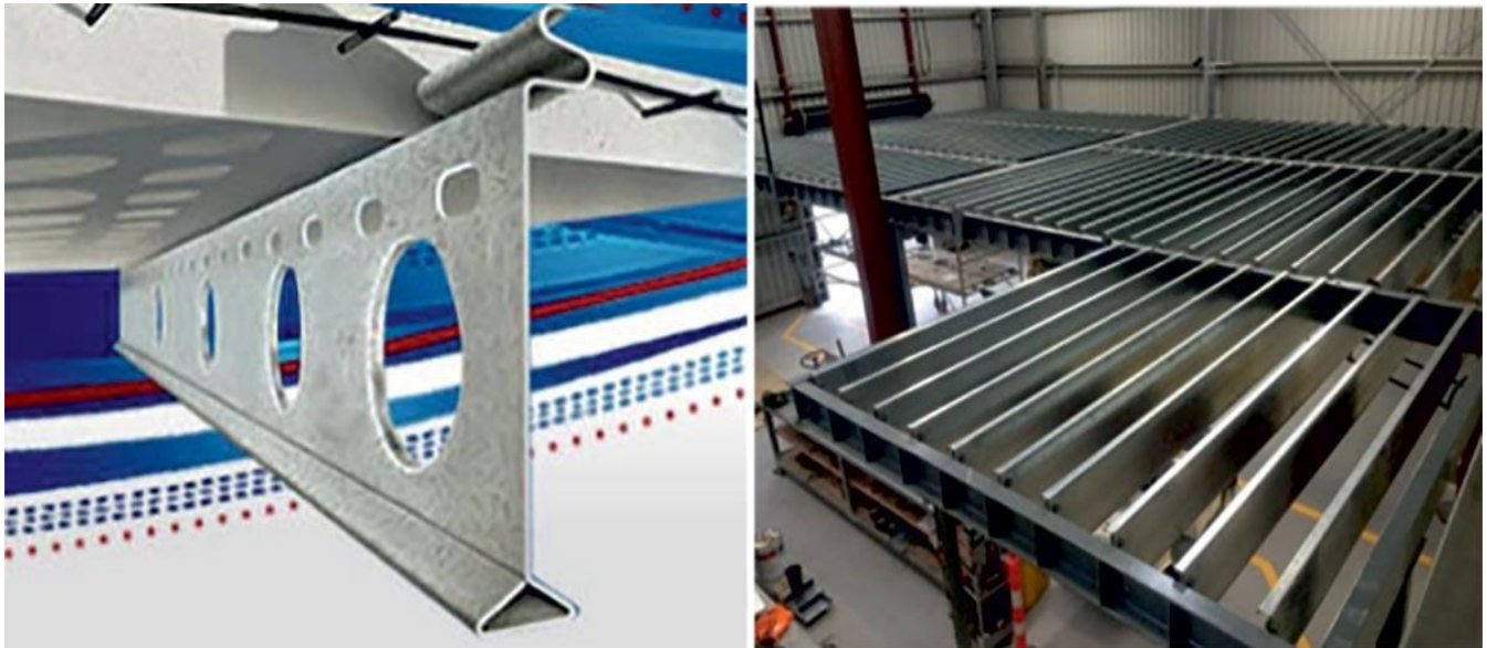
Figure 15: Speed floor system
